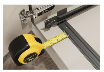
**3.** Measure a minimum distance of 30mm from the edge of the cabinet to the frame.
