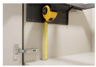
4 Measure a minimum distance of 200mm from the cabinet bottom to the edge of the frame.
